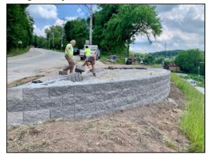
Work has continued at the **Penn Avenue and Lincoln Highway intersection** where the earliest transcontinental roadways have intersected since 1913. The Lincoln statue monument area has been completely reconstructed with a massive retaining wall to ensure total stability of the hillside.
