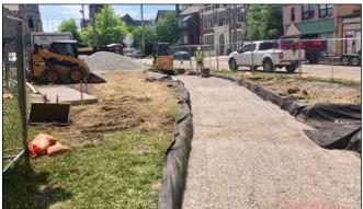
Crushed stone is part of the foundation for the permeable walk to be installed next.
