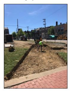
Preparations are made for a semipermeable walkway in the new park. Storm water is managed better with permeable walks.
