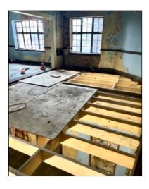
The school entrance ceiling sustained significant water damage. Now the ceiling and floor above it are replaced and the area stabilized. For the first time in a decade or more the building is dry and protected from additional rain. Now we're onto a new flat roof and solar panels. CfCA has received capital funding from the State Historical and Preservation Office, the Hillman Foundation, and an anonymous donor.
